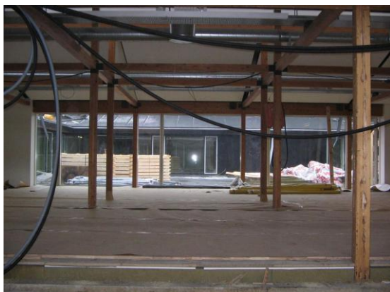
Foto: Renovation of Centre 2 - office area facing one of open gardens. The old wooden structure and the new ventilation system will be part of the visual architecture in the new building.
