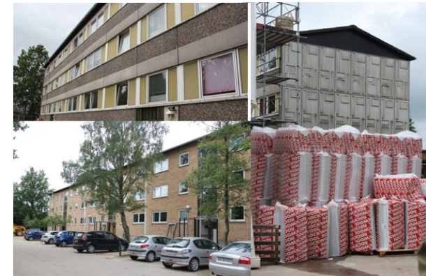
Facades – before and after:
