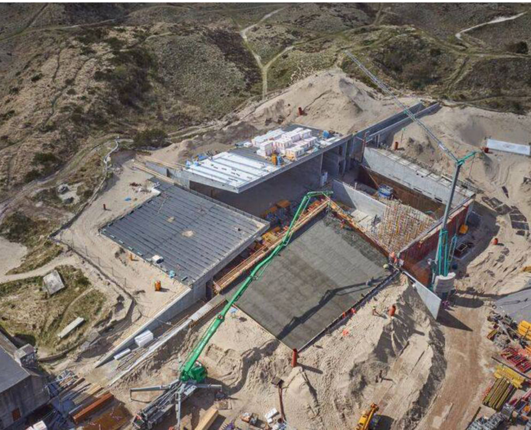
TIRPITZ UNDER CONSTRUCTION & ROOF FORMWORK
